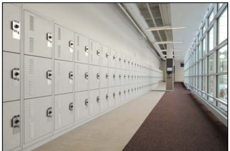
Forty-seven lockers with combination locks designed specifically to store gear bags were installed for the officers use after each shift.
